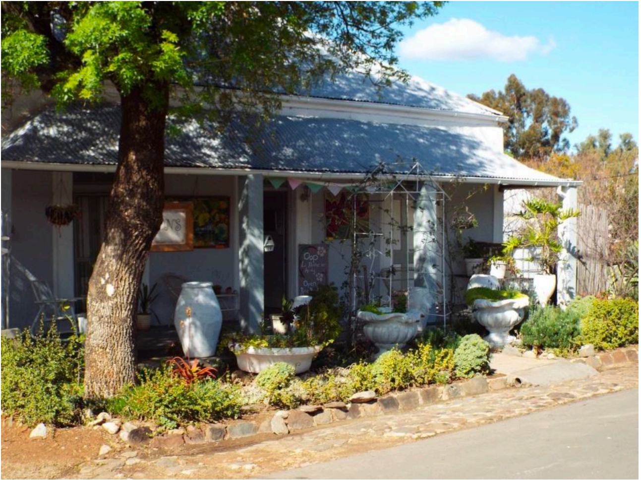
The “Ou Koshuis” in Hoop Street: The old boarding hostel has recently been spruced up as it was in a very run-down condition. This building has not been a school hostel for many years and is now an Art Gallery and residence.
